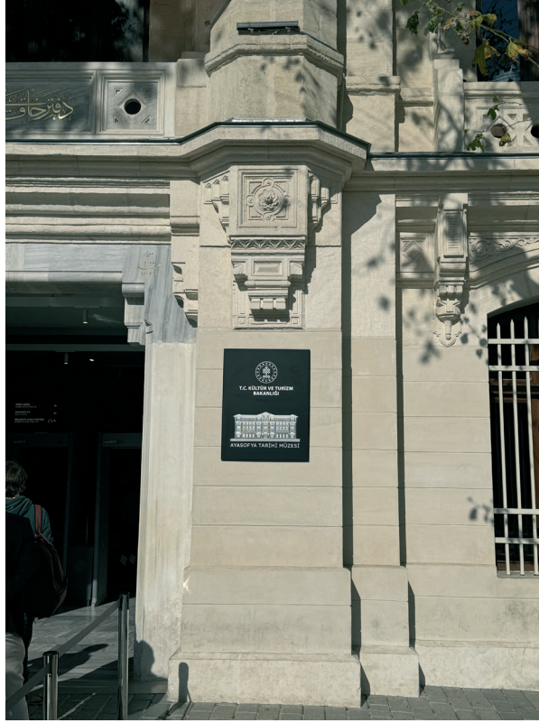
Figure 15. Istanbul, detail from the former Imperial Offices of Land Registry. The ground floor is clad with artificial stone until the arch level of the windows. Above that level is stone-clad. (Photograph: Courtesy of Kadir Ekinci, 2024)
