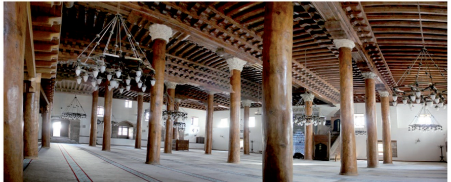
Figure 14. Interior space of Aslanhane Mosque; Wooden structure and Greco-Roman column heads; Perspective by Fevzi Yalım, 1964 (Çelik, Kocabıyıköğlu, 2019); Photo (Author, 2023).
