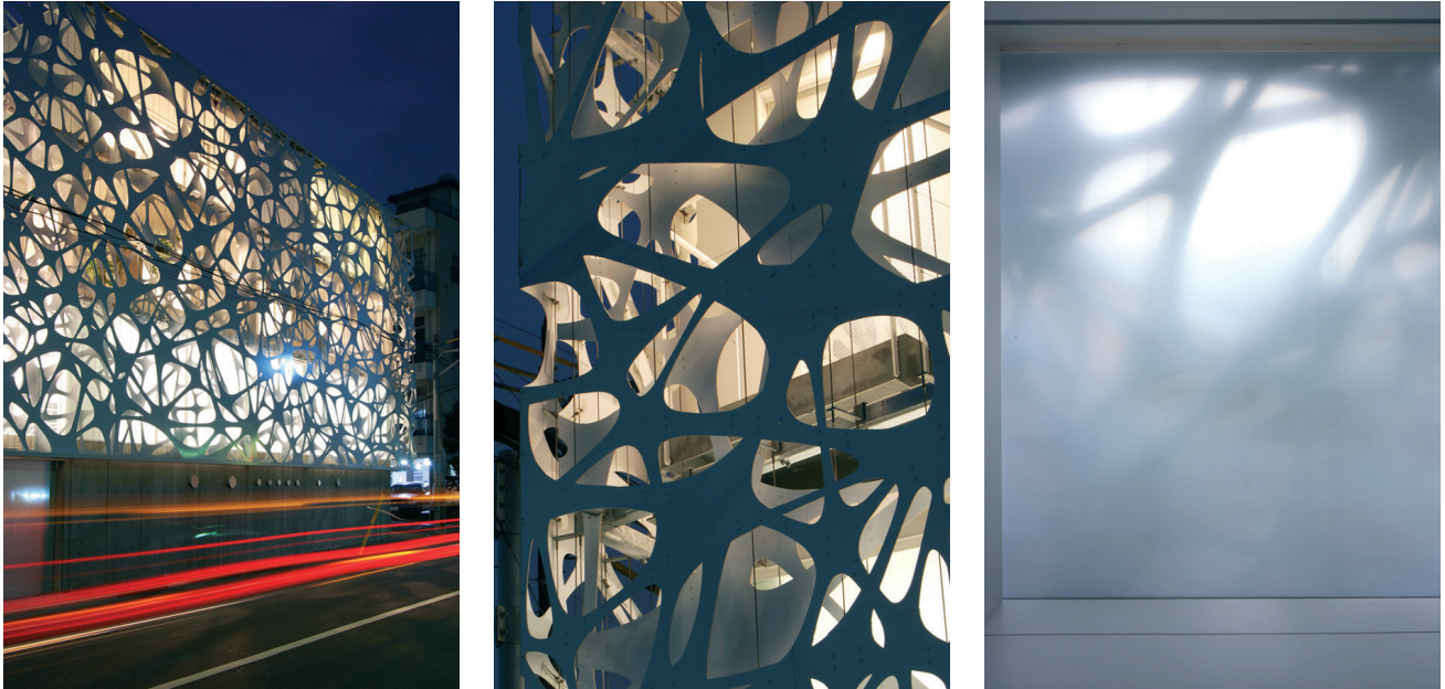
Figures 9a, 9b, 9c. Thom Faulders, Airspace Tokyo, 2007, (Source: Thom Faulders). The façade design is an example of irregularity and customized mass production of singular elements.
