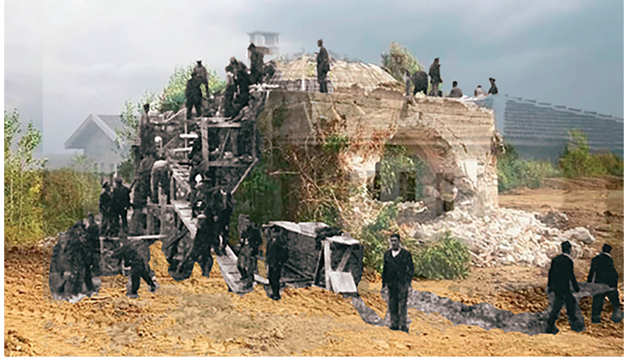
Figure 16. The bathhouse ( hamam ) in Arifiye Village Institute – Photo collage with two photographs of the 1940s and 2018 (Area 2)
