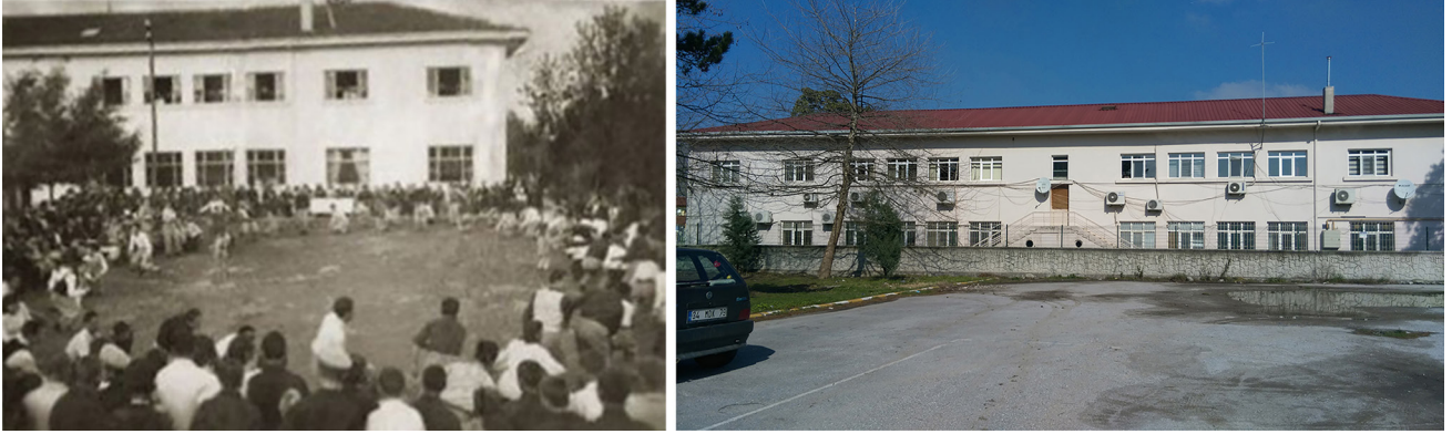
Figure 11. A view of the central classroom building from the area used as a square during the institute period (Karabey Aydoğan Archive; Savaş Archive).
