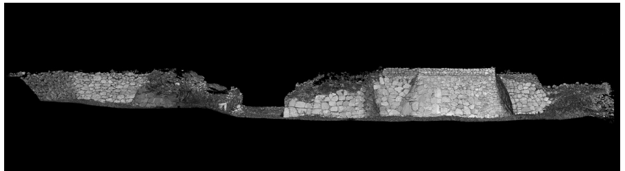
Figure 11. Orthographic image of the Cappadocia Gate: South Elevation. The images were produced by M. Çıngı Salman, Doğan Tekin and Nurçe Düzalan Salman from 3D laser scan data in 2019-2021. (Image: Kerkenes Project)
