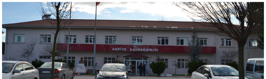
Figure 10. The instructor course's students built the central building in Area 1 (Karabey Aydoğan Archive; Savaş Archive).
