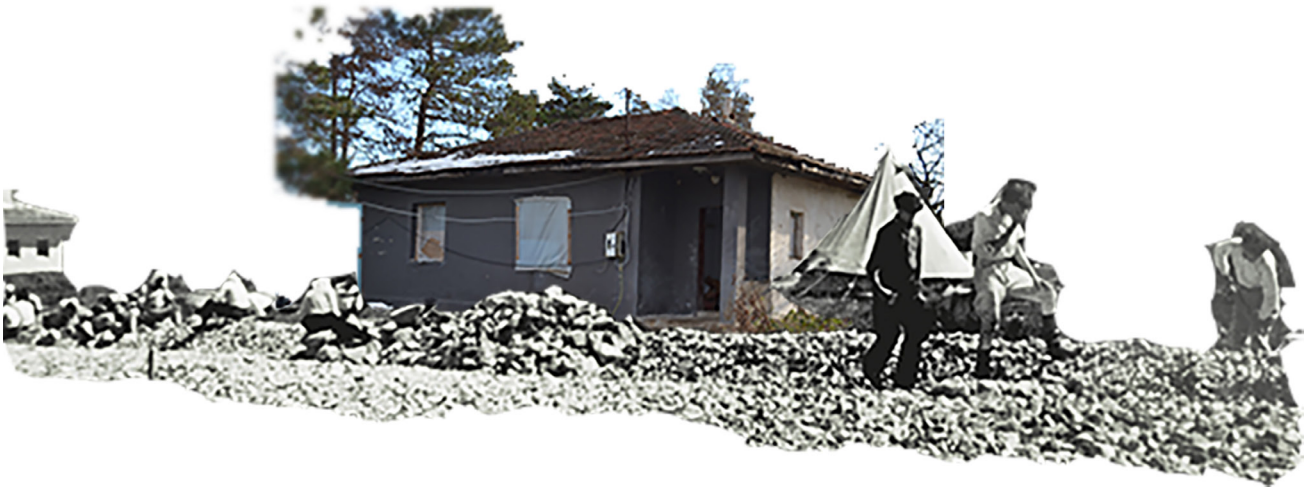
Figure 19. A teachers' house - Comparative study by a photo collage that overlaps a construction period photograph and a 2020 photograph (Area 2)
