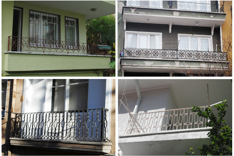
Figure 6. Several balcony balustrades from the research project illustrating ornamental qualities (Tuna Ultav archive)
