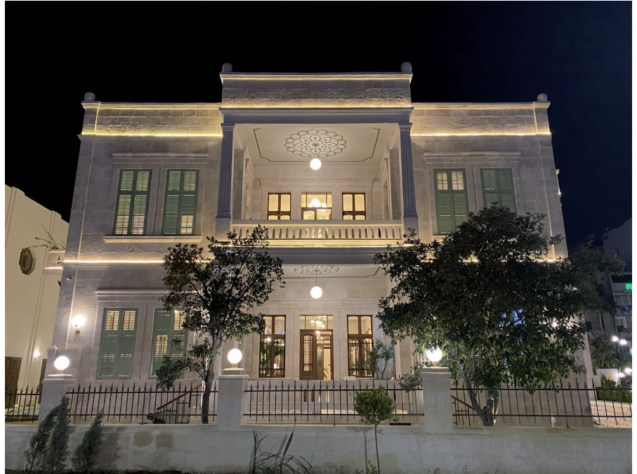
Figure 17. The east façade of the building after restoration (Photograph taken by the author, 2021)
