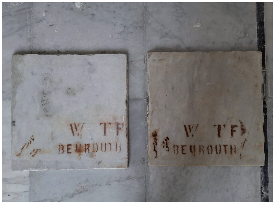
Figure 21. Stamp showing the production location of the marble plates covering of the first-floor slabs (Photograph taken by the author, 2021).
