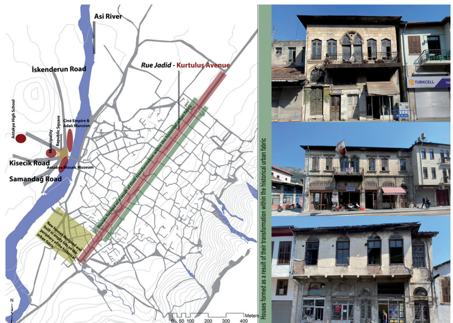
Figure 9. Examples of formed and transformed houses on the Kurtuluş Avenue (Prepared by the author, 2020).
