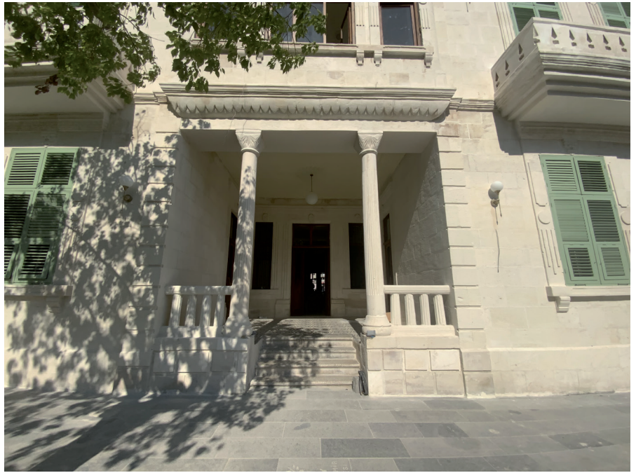
Figure 16. The entrance of the west façade (Photograph taken by the author, 2019).
