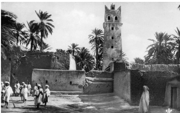
Figure 10. Minaret of the Sidi Ben Fadhel mosque (Photographes De Biskra, n.d.)
