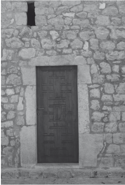
Figure 38. Clock tower's entrance door, 2018 (Photo by R. Alihodžić).
