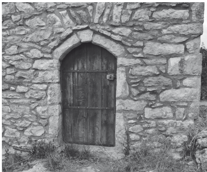
Figure 33. Clock tower's entrance door with a Tripartite Stone Arch, 2018 (Photo by R. Alihodžić).
