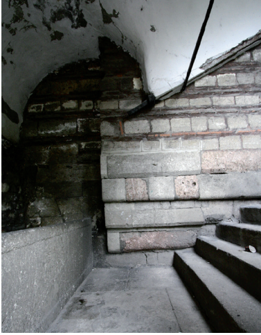
Figure 13. Northwest Façade, Type F Wall Masonry View from Staircase, 2012.
