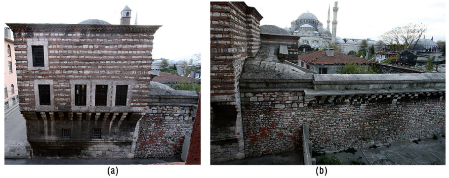
Figure 19. (a) Northeast Façade, (b) Garden Wall and Load-Bearer Stone Projections, 2012.
