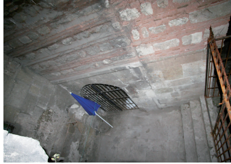
Figure 15. Northeast Wall of the Semi-Open Space Indicating the Difference in Masonry, 2012.
