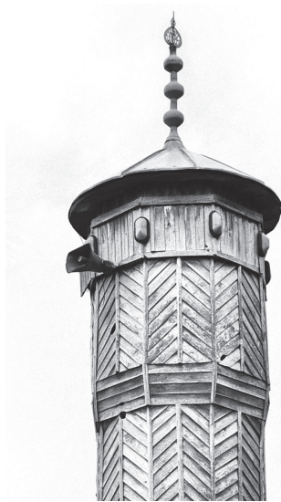
Figure 12. The Minaret of the Atik Mosque (Photo by E. Jahić)
