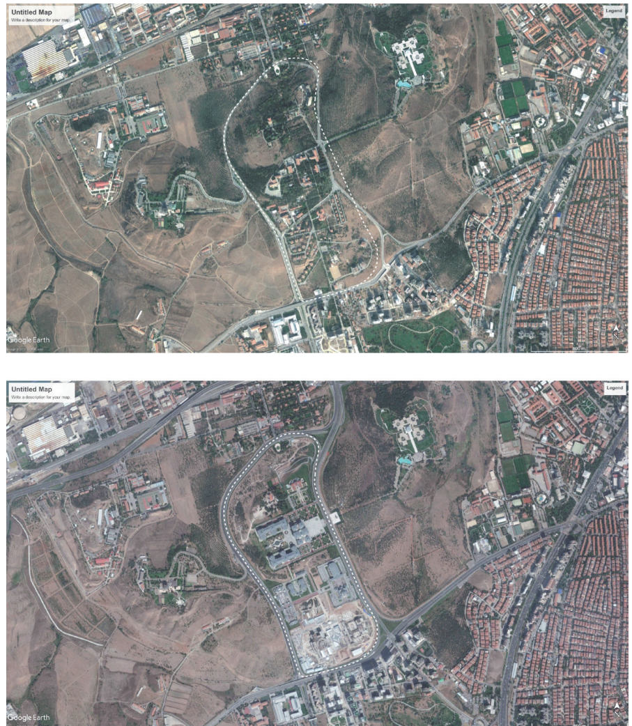
Figure 1. Boundaries of the “Turkish Republic Prime Ministry Gazi Settlement Urban Transformation and Development Area” in 2009 (top) and 2017 (bottom) (Source: Official Gazette, 2012/3074)
