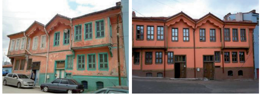
Figure 2. A historic house in Odunpazarı, province of Eskişehir. Before and after restoration. Source: Ministry of Culture and Tourism
