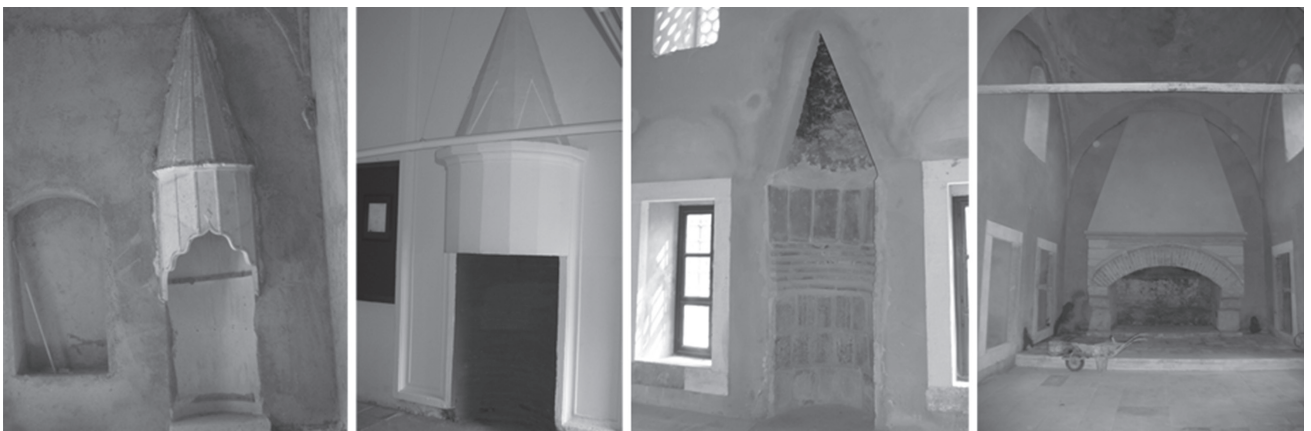
Figure 18. Fireplaces in Haseki (left), Bayezid II (middle-two), and Süleymaniye (right) Hospitals (Photos by the authors, 2011).
