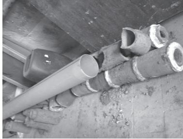
Figure 4. Terracotta pipes unearthed on the passage between Sivas, Izzeddin Keykavus I Hospital /Şifahiye and Çifte Minareli Medrese, found in situ at the foundation wall level of the medrese and stored inside the entrance ıvan of the hospital during 2011 restorations (Photo by the authors, 2011).
