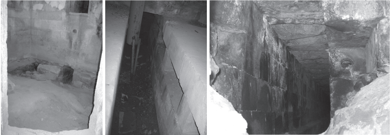
Figure 10. Caldarium of the bath section showing hypocaust channels in Doğu Bayezid, Ishak Pasa Palace (Photo by the authors, 2012).
