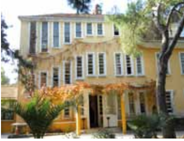
Figure 23. A detail from the Spa Hotel (S.Ateş archive, 2011).
