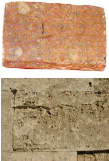
Figure 4. Maetra Sarmatimactra from Pınarhisar quarries on left (Küçükaya 2004) and fossil limestone used on the wall of Sultanahmet Mosque in İstanbul.
