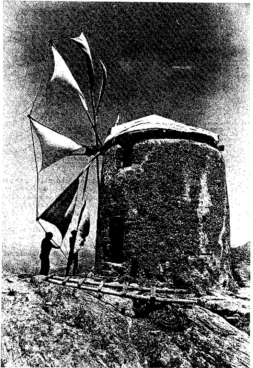
Fig. 22 The miller and a farmer roll up the canvas of the sails to close the mill after a session of grinding.
