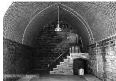
Figure 12a, 12b. An under ground ice house (left) and its plans and sections (right) in Orumie (Ghobadian, 2001).
