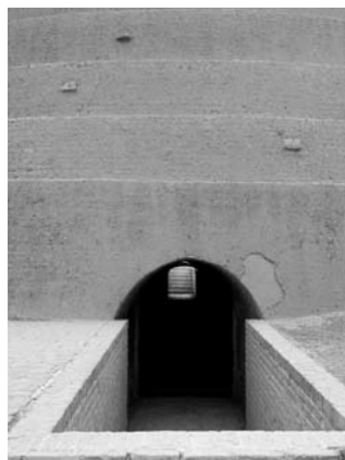
Figure 10a, 10b. Figure 10a shows a southern entrances of an ice house which was used by the person in charge, and the 10b looks through the inside of an ice house which stairs and sloped surfaces are designed to help man and ice transfer (Andrew Schnider, 2010).
