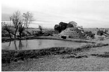
Figure 7. Alaghbeig ice repository without the shading wall with its great pool in front of it ( Hosseini, 2011).
