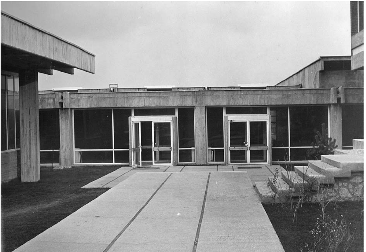
Entrances to Department of Civil Engineering, KI.
