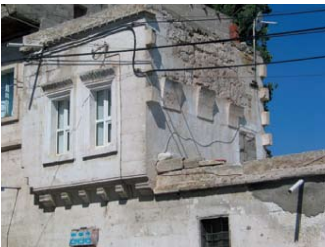
Figure 17. Unfinished stone masonry construction expressing sustainable/ open-ended construction or additive quality of buildings.
