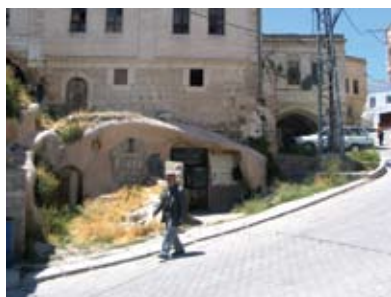
Figure 18. Old laundry now used as a Slaughterhouse.
