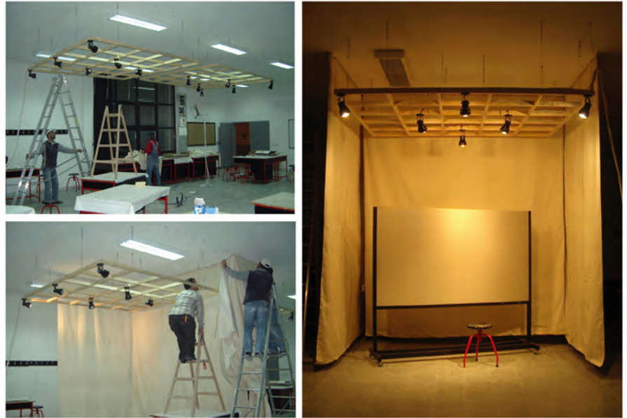
Figure 1. The mock-up application; Left top and bottom: Construction process of the mock-up application; right: one of the two design spaces defined by the mock-up enclosure (2 x 3 x 3.5 meters).
