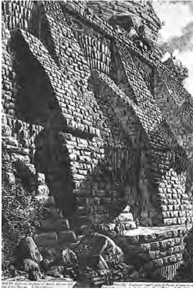
Figure 21. Foundations of Hadrian's Mausoleum (later Castel Sant' Angelo), Le antichità Romane , IV, 1756.
