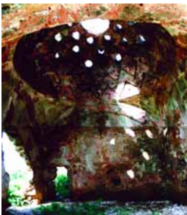
Figure 23. Oruç Paşa Hamam , Didymoteichon. The disrobing room and its entrance. The rhombic patterned dome with the oculus (E. Kanetaki).
