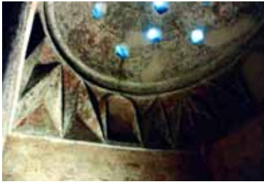
Figure 21. Bey Hamam , Thessaloniki Turkish triangles in a halvet dome (E. Kanetaki).
