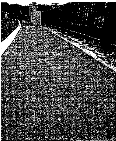
Figure 5. Fly ash from municipal incinerators is used to make these bricks (ENV, 1997d, 26).
